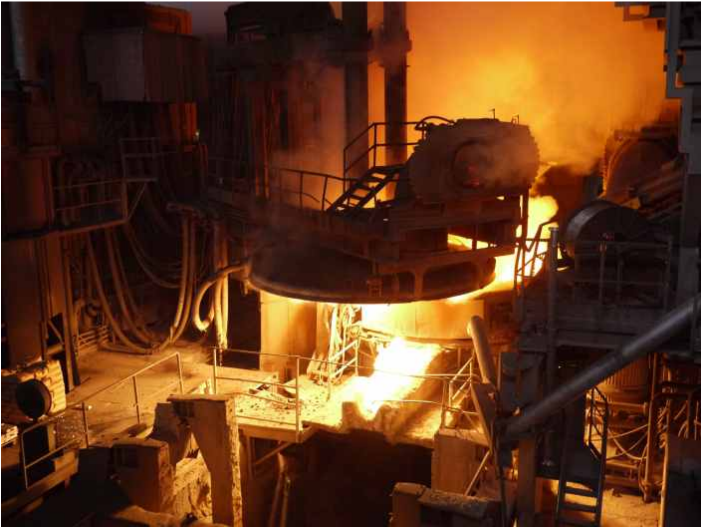
Above: a lift and a move of the EAF's arch before loading of the furnace with scrap
