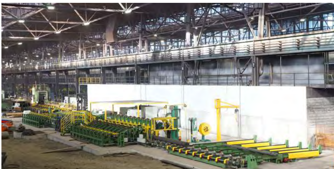
Above: new foreman's office, below: new control line for round profiles
